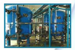
impurity ions present in the water are replaced by ions released by an ion-exchange resin. The impurity ions are taken up by the resin, which must be periodically regenerated to restore it to the original ionic form. (An ion is an atom or group of atoms with an electric charge. Positively-charged ions are called cations and are usually metals; negatively-charged ions are called anions and are usually non-metals).
