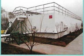
Multi Stage Biological Treatment system is an advanced and highly efficient method of treating industrial and municipal waste water. Multi Stage Biological Treatment (MSBT) is an efficient method of domestic and industrial wastewater treatment based on spatial microorganism's succession and trophic hydrobiontchains.
